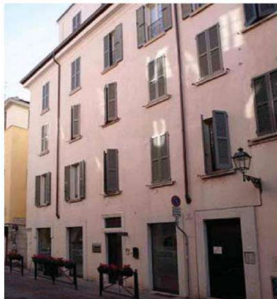
Figure 2 - Via del Carmine 15 building- Immobiliare Sociale Bresciana for single mothers and single women.
